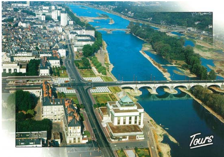
Figure 9 City Library, Tours, France
