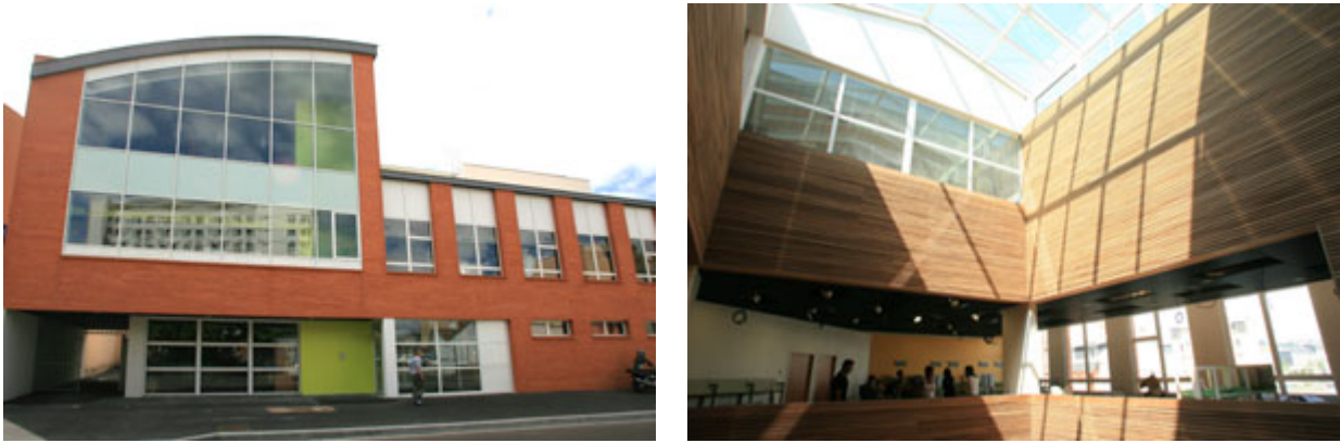
Two views of the new library at Le Havre France
