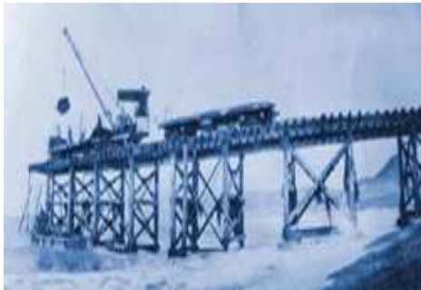
Crane unloading passengers to the dock
